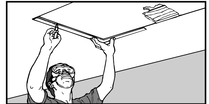
Figure 9 Draw a rectangle the size of the rough opening.
